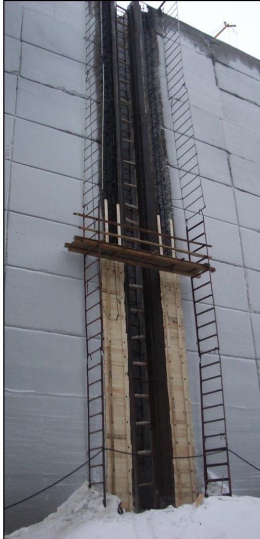
3) Casing and concreting
