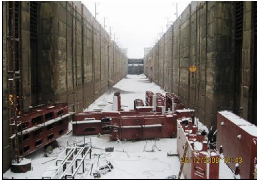
Mounting of new gates
