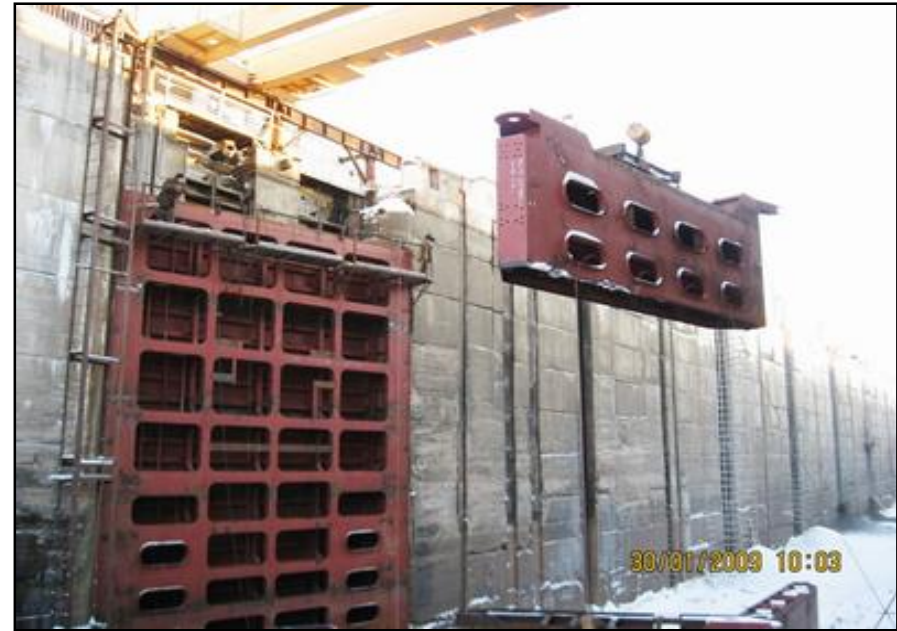
Mounting of new gates
