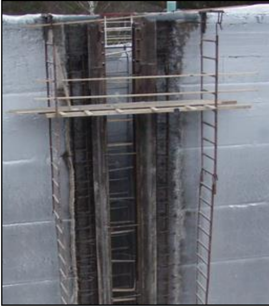
2) Reinforcing of concrete
