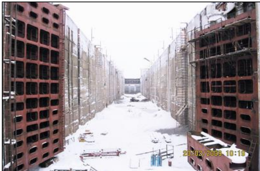
Mounting of new gates
